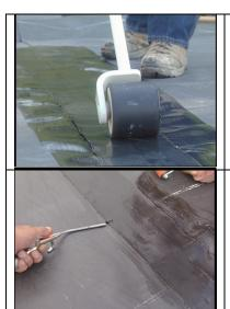
**Step 6**- Using either a hand or stand-up roller; roll the seam longitudinally and across the seam in overlapping sections to mate the seam together.
