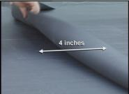
**Step 2**- Overlap the adjacent PondGard panels by a minimum of 4". Allow the PondGard panels to relax for 15 minutes.
