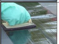
**Step 3**- Using a scrubber pad and holder; apply the QuickPrime Plus primer to the top surfaces of the adjacent PondGard panels covering a minimum of 4" on both sides of the overlap edge.
