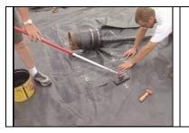
**Sub Step 4**- Seam the target patch to the PondGard panel with primer and either 6" QuickSeam Cover Strip or QuickSeam Splice Tape (See either Detail 9- Creating A Seam With 6" QuickSeam Cover Strip Tape or Detail 10- Creating A Seam With 3" QuickSeam Splice Tape).
