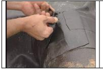
**Step 3**- Once the PondGard is properly positioned over the pipe adhere a piece of QuickSeam FormFlash to the pipe.
