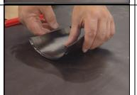
**Step 4**- Install the QuickSeam patch by peeling away the release paper and placing the patch over the damaged area of the liner.
