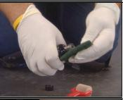
**Step 2**- Apply the QuickPrime Plus primer by pouring a small amount onto the scrubber pad and applying it to the surface of the PondGard beyond the perimeter of the area to be repaired with a patch.
