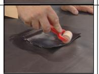
**Step 5**- Roll the patch evenly over the area to be repaired in order to properly mate the patch and liner together.
